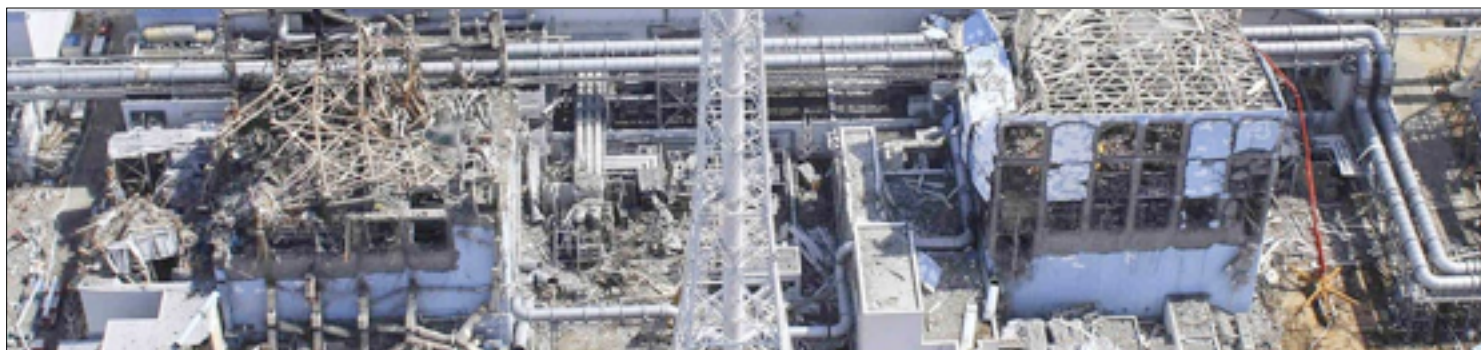
Fukushima units Nos. 3 (left) and 4 on 24 March 2011, looking seaward. No. 3 is in meltdown. No. 4's 90 metric tons of fuel rod assemblies (about 60 tons of uranium oxide and isotopes) had joined 130 tons of older "pins" in the 5th floor spent fuel pool during reactor maintenance. A hydraulic cement pumping truck (red pipe) is trying to replace the boiled off water in the pool. At 1200 deg C, the fuel rods oxidize directly with the remaining water's oxygen, leaving hydrogen gas explosions to cause the visible damage. Unmanned aerial drone photo released by Air Photo Service.
